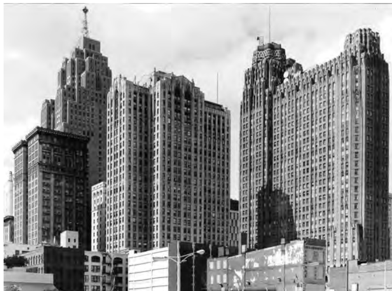
Architecture in Detroit
