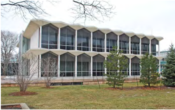
McGregor Memorial Conference Center, Wayne State such as those found in the Guardian and Penobscot buildings.
