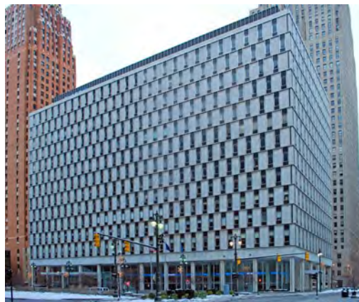
National Bank of Detroit Building
